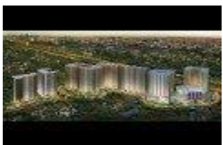
(13) Bassura City (Jalan Basuki Rahmat)
