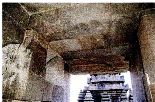
Cracks on the outer wall and alley of west gate way of Siwa Temple.
