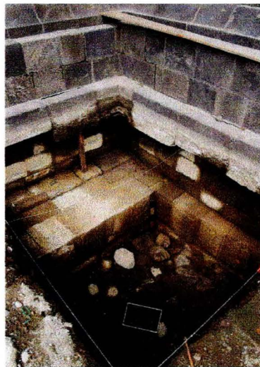
Excavation on Siwa Temple
