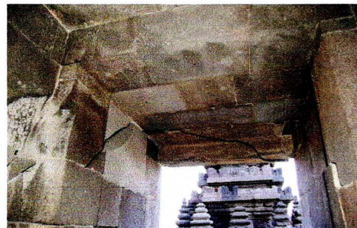
Cracks on the outer wall and alley of west gate way of Siwa Temple.
